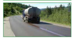
CRF® Restorative Seal is a cationic blend of asphalt and rejuvenator applied to pavements that exhibit more moderate deterioration including increased raveling, loss of aggregate and minor alligator cracking. Providing a "seal in depth," CRF® Restorative Seal is flexible and resilient.
