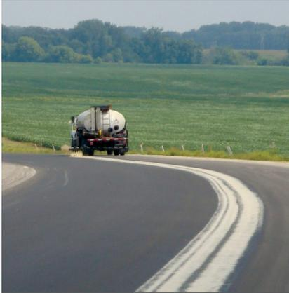
JOINTBOND Being Applied to Longitudinal Joint Area
