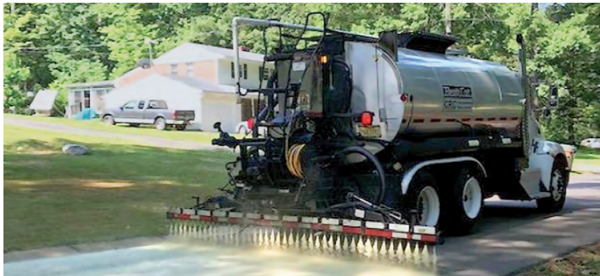
PlusTi A.R.A.-1 Ti® asphalt rejuvenator/sealer application
