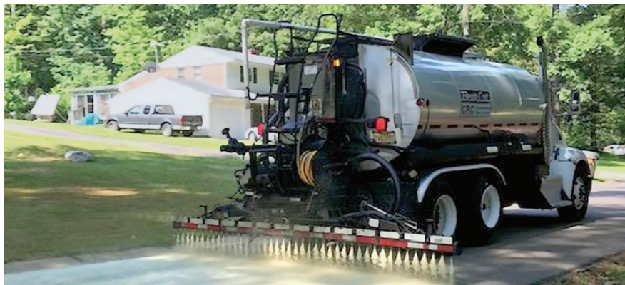
PlusTi A.R.A.-1 Ti® asphalt rejuvenator/sealer application
