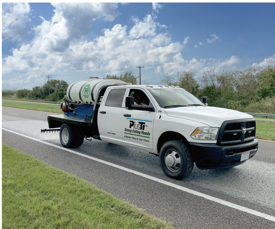
PlusTi Ti-intro CME penetrant application
